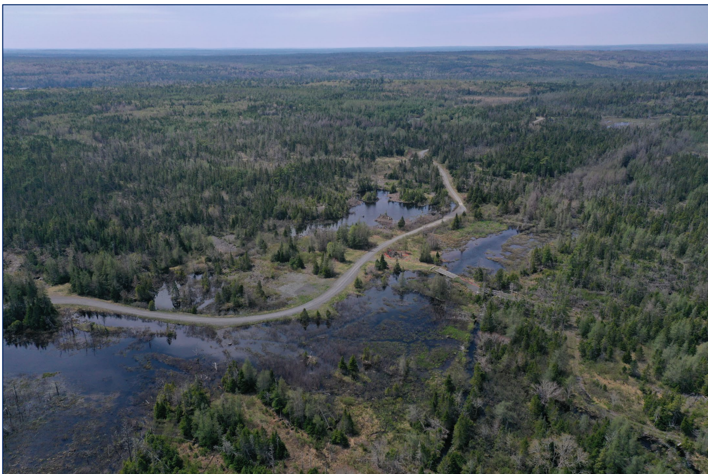
Figure 2: Existing historic 15-Mile project site
